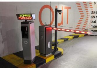
Basically, the Boom barrier gets an open/close signal from LPR, but can also be controlled using manual switch from the managing center if required.
