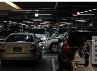
Then drivers can find available parking bays easily by checking the color of LED indicator (Green: Available / Red: Occupied)
