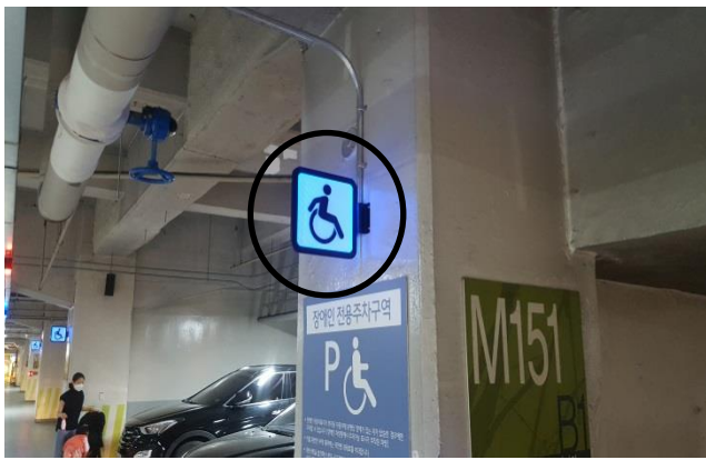
LED Indicator for handicap parking spaces
